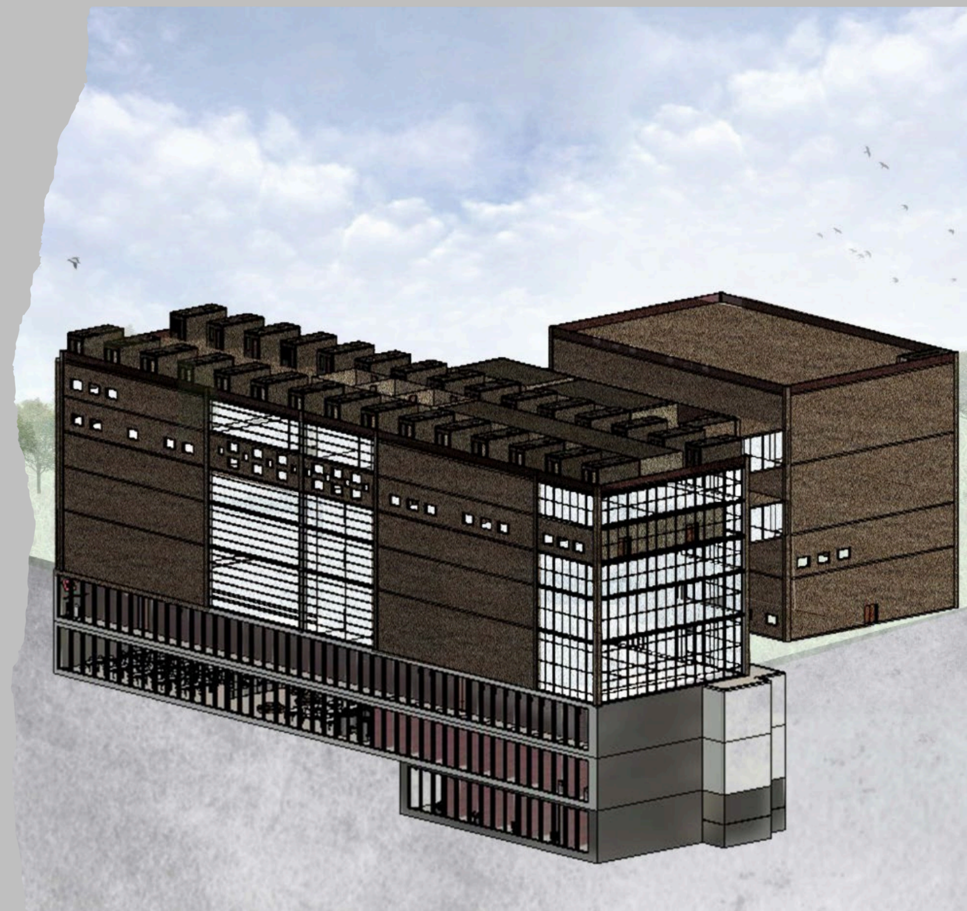
Perspective View: The architecture of the building optimizes cross-ventilation between the two sides through extensive use of louvers and natural lighting through exterior glazing.
