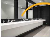
Sink system integrated with mirrors and soap dispensers (DfMA)
