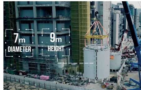
The MiC thermal tank weighted 50 ton each being just-in-time installed to the site. Image Courtesy of Global Switch
