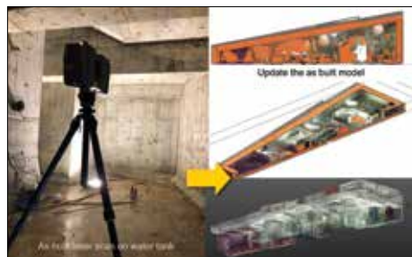
As-built BIM Model updated based on as-built laser scan data for proper documentation. Image Courtesy of Urban Renewal Authority
